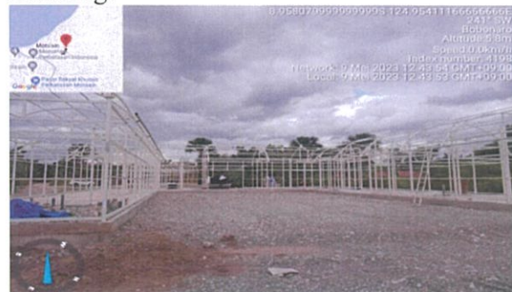
Foto : Rangka kuda – kuda ba Dormitory Building.
