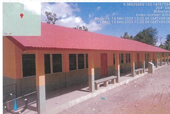
Foto : CLASSROOM BUILDING C
