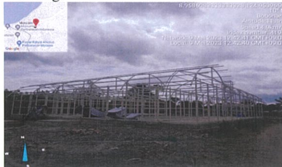
Foto : Rangka kuda – kuda ba Dormitory Building.
