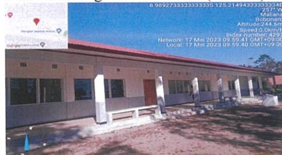
Foto : Building Teacher Office (exterior).
