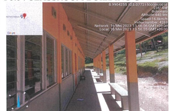
Foto : CLASSROOM BUILDING C
