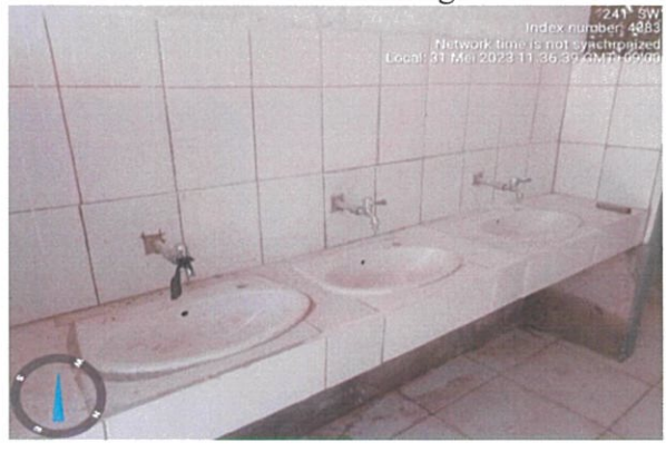
Foto : Assessoris Toilet Building Tb
