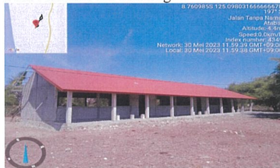
Foto : Classroom building C.
