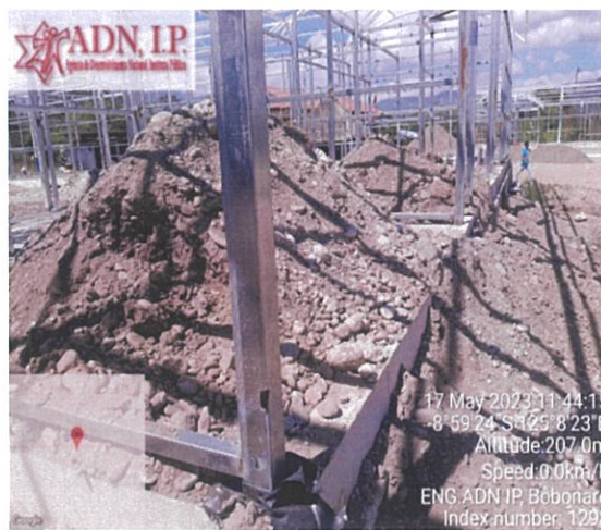
Foto ; Column Hollow steel 80x80mmx2mm for Dormitory Build.
