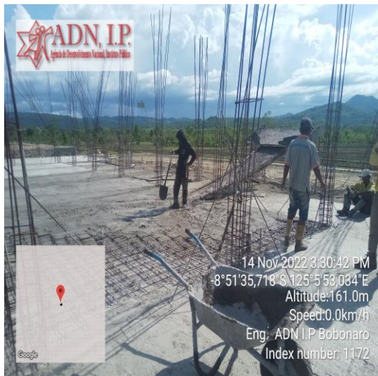
Foto : Kontinua pengecoran lantai ba Building Dinning Hall & Kitchen
