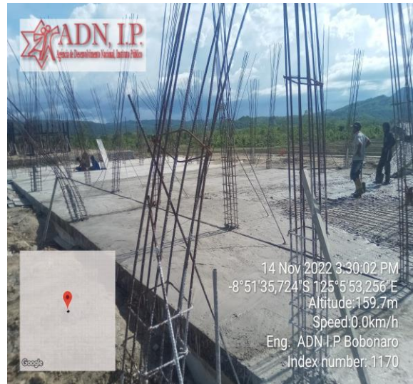
Foto : Kontinua pengecoran lantai ba Building Dinning Hall & Kitchen
