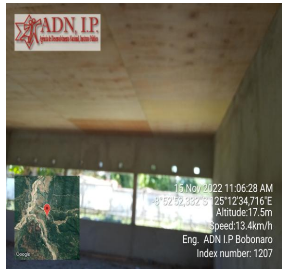
Foto : Class Room Building C (Parte Interior).
