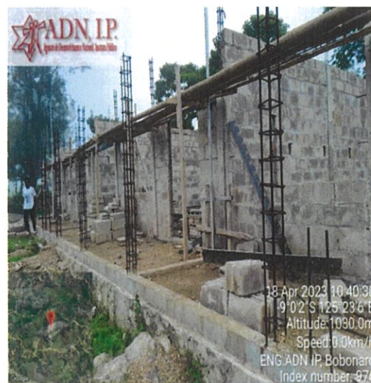
Foto : Servisu pembesian colom building Classroom.
