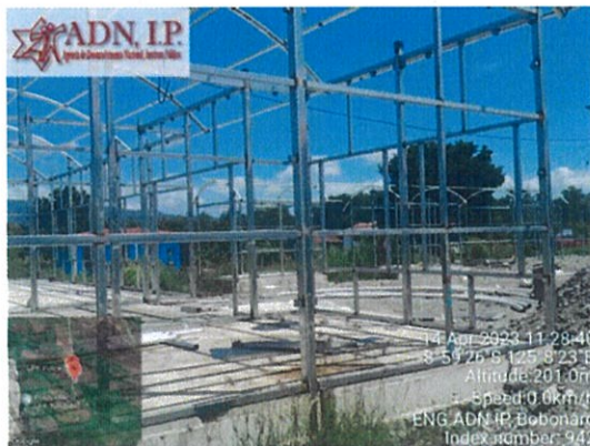
Foto : Servisu rangka dinding hollow steel uk 50x50mmx2mm for office building
