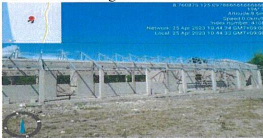
Foto : Servisu monta kuda – kuda classroom building C.
