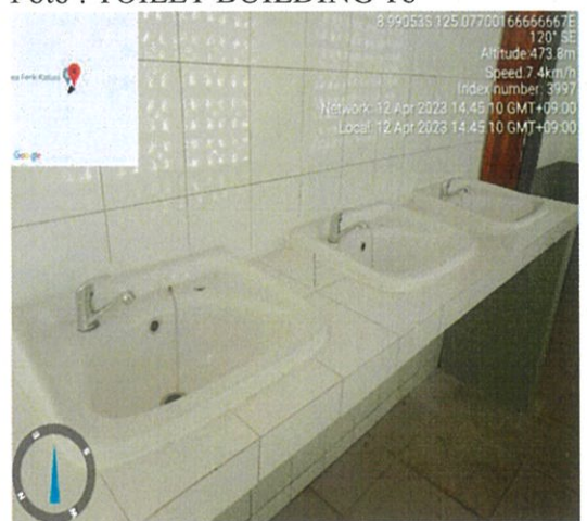
Foto : TOILET BUILDING Tb
