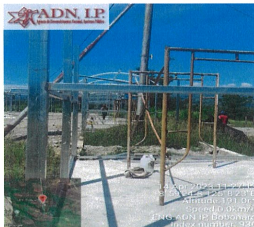
Foto ; Column Hollow steel 80x80mmx2mm for Post Build.
