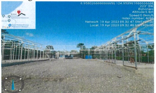
Foto : Rangka kuda – kuda ba Dormitory Building.
