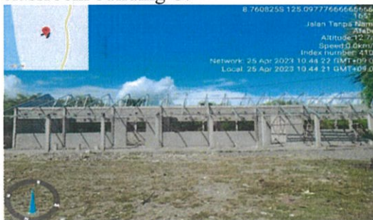
Foto : Servisu monta kuda – kuda classroom building C.
