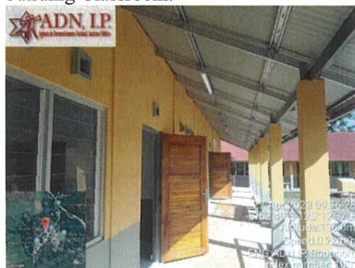
Foto : Servisu pemasangan daun pintu building Classroom.
