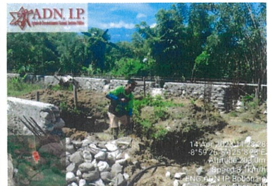
Foto : Servisu fondasi building meeting room
