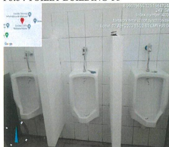
Foto : TOILET BUILDING Tb
