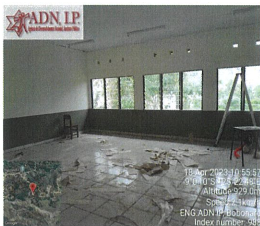
Foto : Servisu pemasangan keramik 400x400mm building Classroom.
