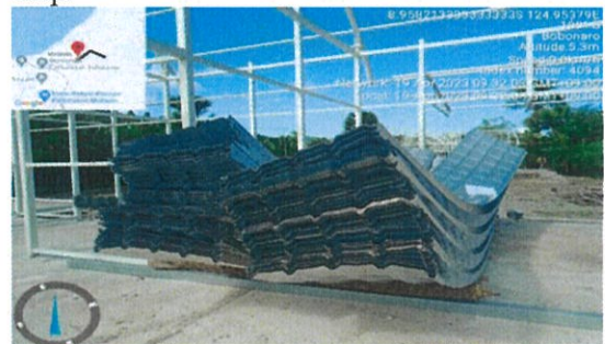
Foto : Material on site kaleng ba servisu atap.
