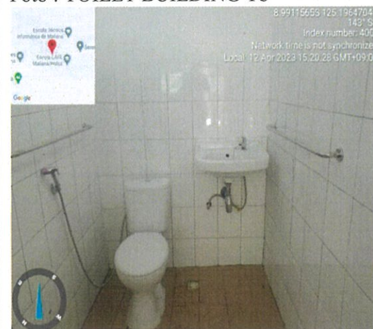
Foto : TOILET BUILDING Tb
