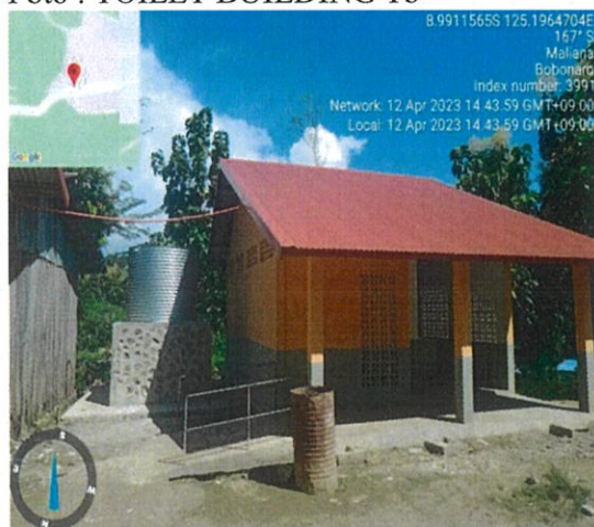
Foto : TOILET BUILDING Tb
