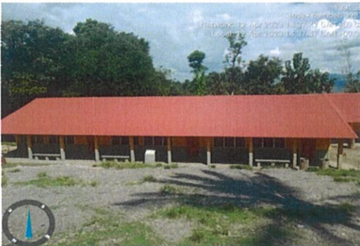
Foto : CLASSROOM BUILDING C
