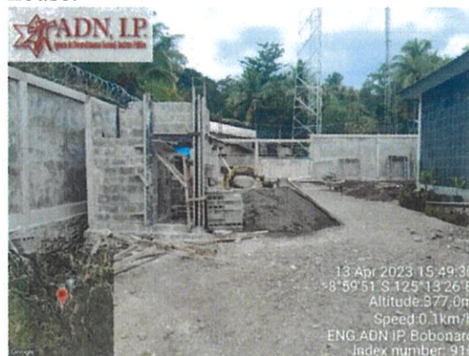
Foto : Servisu bekisting column Guard house.
