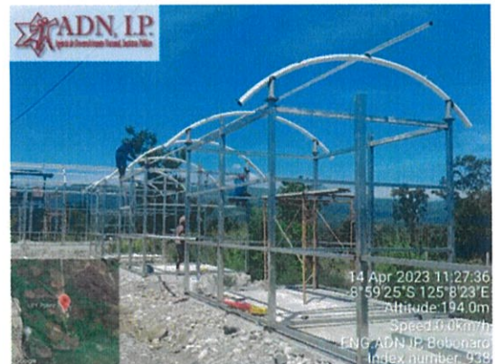
Foto: Servisu Column hollow steel uk 80x80mmx2mm iha office building.
