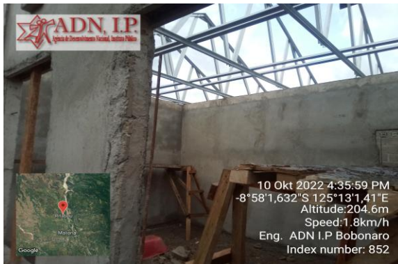
Foto : 15mm render to internal surfaces of internal block walls
