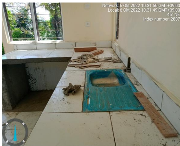
Foto : Servisu monta keramik ba meja beton inklui mos fase bikan / kitchen set ba Building Doctor house.
