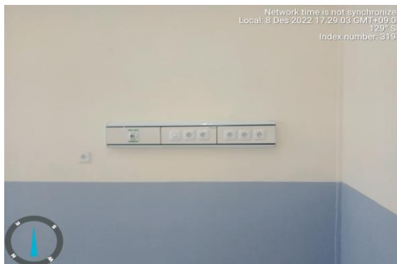
Foto : Supply and install Headbet for outlet/GPO 1450mm AFFL include wall box.
