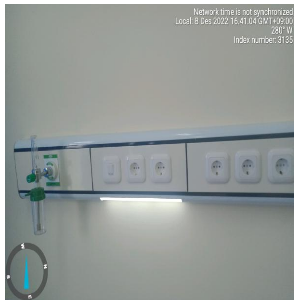
Foto : Supply & install Headbet for Outlet/GPO 1450 mm AFFL include wall box.
