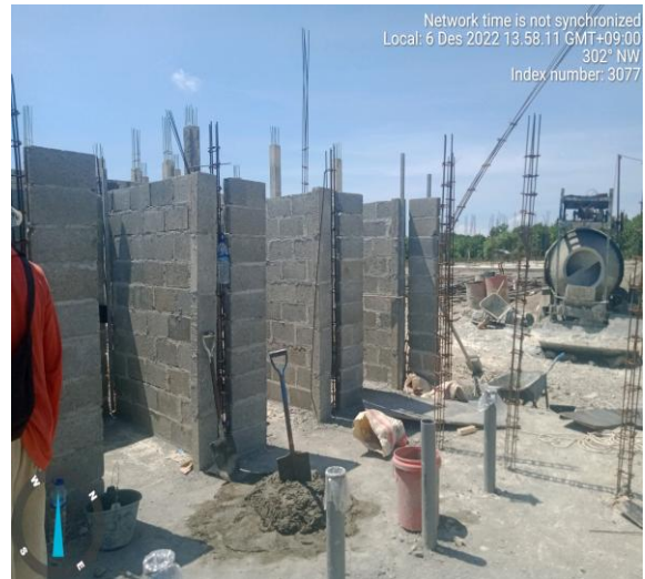
Foto : Servisu monta batako ba area Building Toilet
