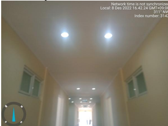
Foto : Supply & install Lighting bold lamp 24 W "Philips"
