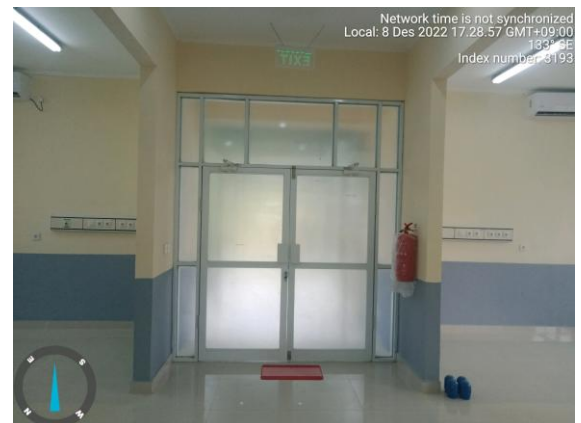
Foto : Supply and install Emergency Exit lamp 10 W
