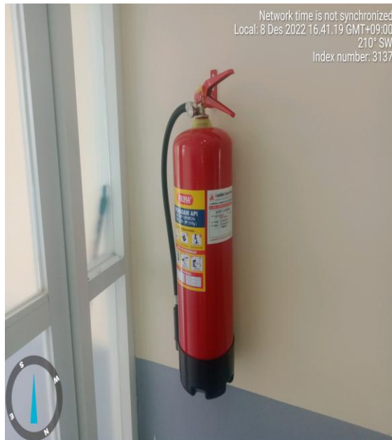
Foto : Supply & install Fire extinguisher 9 kg
