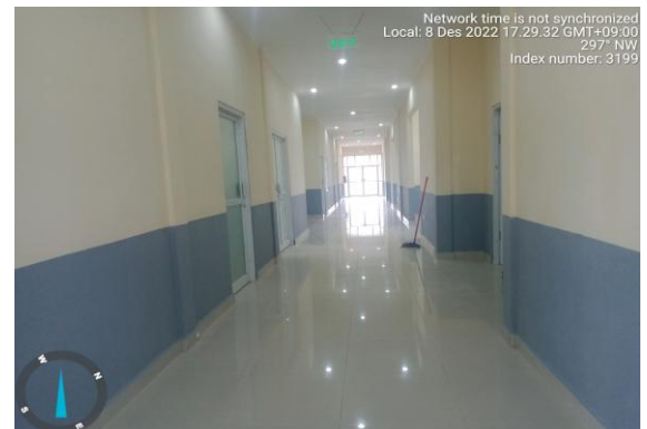
Foto: Supply and install Lighting Phillips F2 hold lamp 24 W
