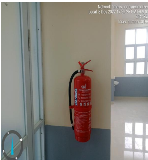
Foto : Supply and install Fire extinguisher 9 Kg
