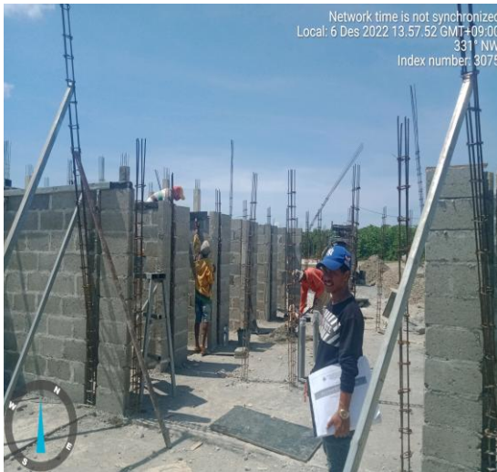
Foto : Servisu monta batako ba area Building Toilet
