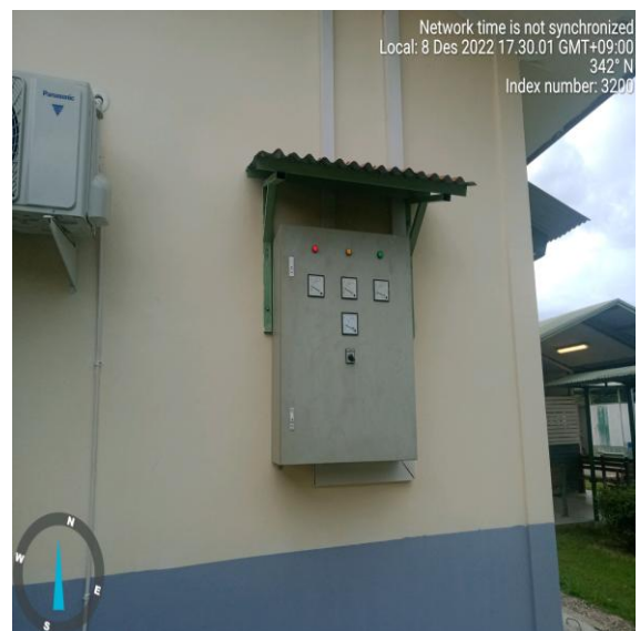
Foto ; Suply and install Distribution Panel Board + all accessories (Inc, connect to EDTL).
