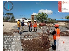
Viqueque, (27/10/) ADN, I.P. UCVQ nia Técnica Edifikaun Munisípiu Viqueque hala'o inspeksaun ba projetu new construction of health post and doctor's house building in Builale-Ossu.
