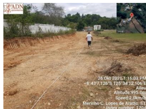
Aileu, (26/10) ADN, I.P. Liu husi UCVQ nia Técnica Edifikaun Munisípiu Aileu hala'o inspeksaun ba projetu new construction of campas gate leveling area in garden of heroes in Aileu.
